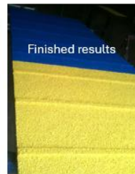
Ramps have contact zones Here the transition is made to yellow (note forms must be removed promptly)
