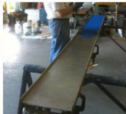
Spread granules on the primed surface With a clean towel (forms are clamped to contain granules)
