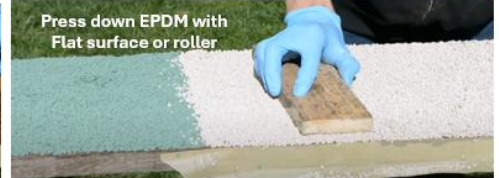
Sprinkle on a Layer of EPDM
